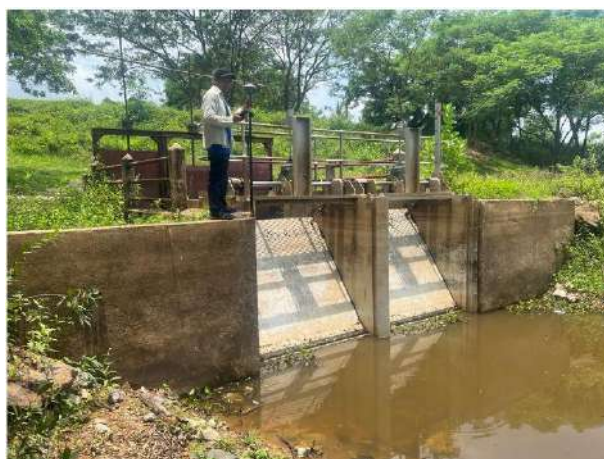
Figure 3-6 Bottom hinged gates at Nong Peung outfall
