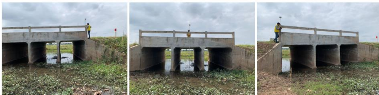
Figure 17: Surveyor was operating RTK rover to measured bridge points
