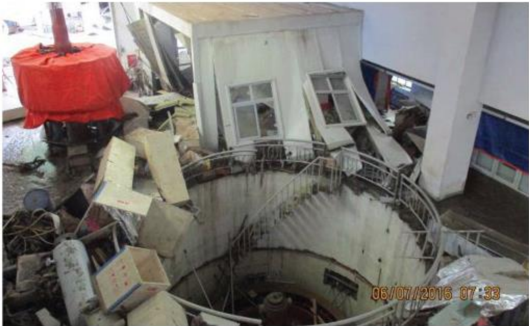
Figure 49. The control room on the erection bay floor was completely destroyed by flooding of the powerhouse (Source: Bruen et al., (2017))
