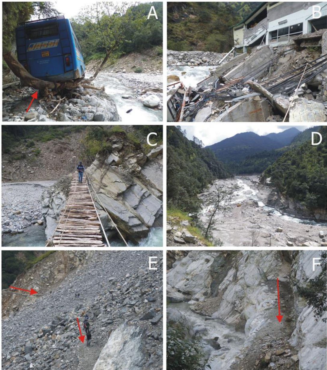
Figure 36. Photographs showing the devastation between Sonprayag and Gaurikund: (a) Red arrow indicates direction of motorable road, which was completely damaged near Sonprayag; (b) power house station, which was entirely smashed; (c) broken bridge site and temporary overpass on the Songanga tributary of Mandakini River; (d) downstream flood-affected view of Sonprayag; (e) damaged road between Sonprayag and Gaurikund; red arrow shows direction to Rambara, and (f) flood level of Mandakini and damaged road near Gaurikund; red arrow shows direction to Rambara (Source: Bhambri et al., (2016)).
