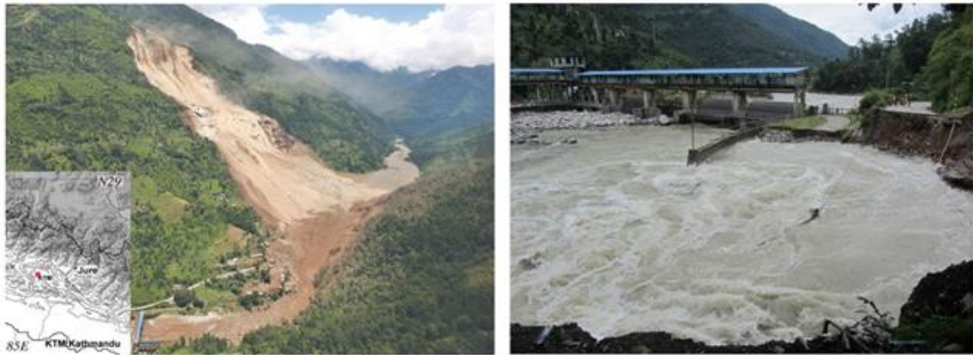
Figure 39. Jure landslide on the Sunkoshi River (left). Damages to Sunkoshi hydropower and Araniko highway after the breach of the landslide dam (right) (Source: Retrieved from Google on 15 th July 2021).
