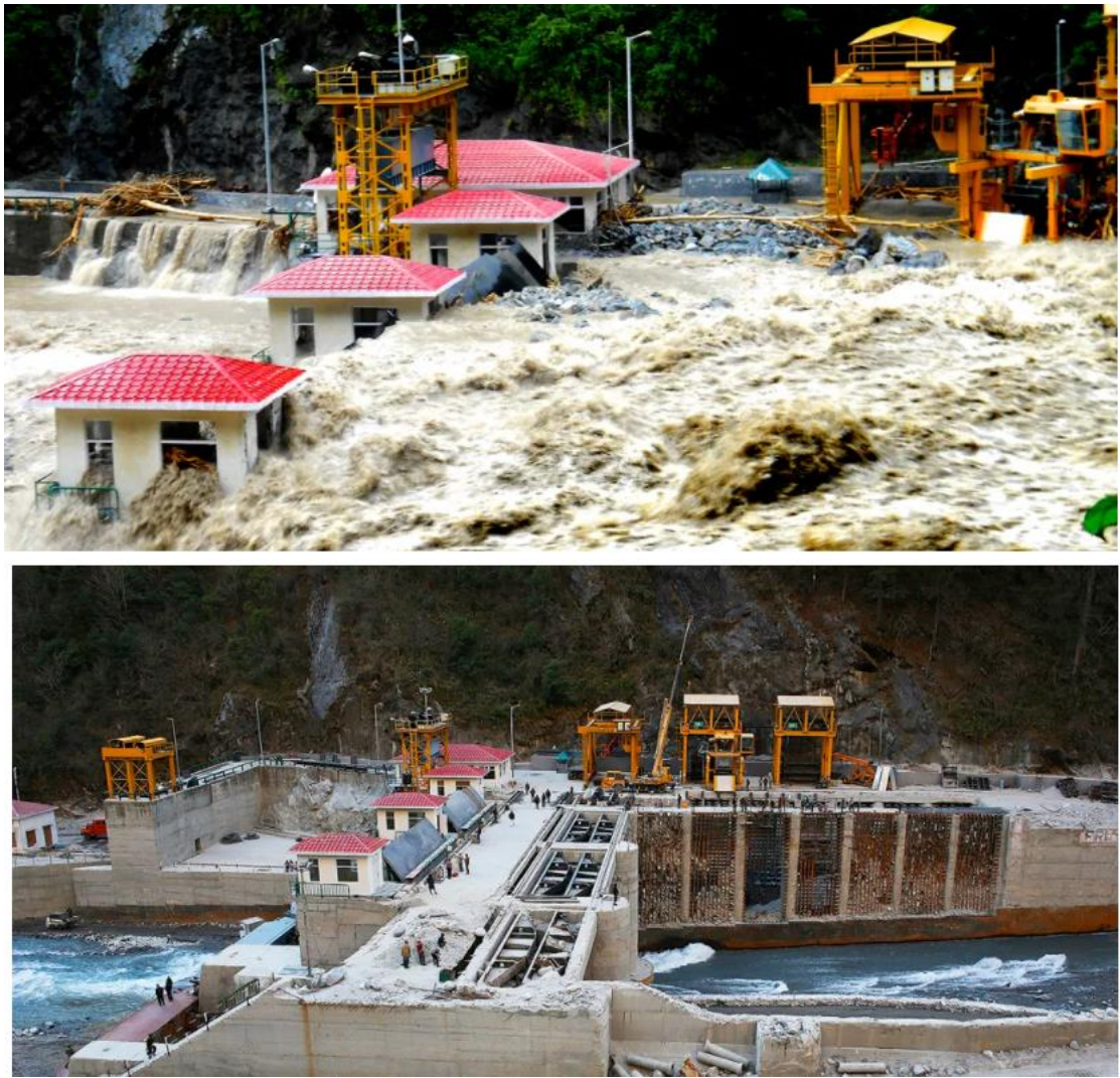
Figure 38. The Uttarakhand flood exceeded every previous high-end boundary of water surge, infrastructure failure, and survivability. At the Vishnuprayag Hydroelectric Project on the Alaknanda River, floodwaters surged over the 55-feet tall dam and boulders buried it in 60 feet of rubble. (top). Mud and silt still lie in piles on the top of the dam. The cracked and ruptured concrete, and exposed steel reinforcing bars on the dam's walls, are evidence of the beating the dam took from the Uttarakhand flood in mid-June 2013 (bottom) (Source: https://www.circleofblue.org/ ).
