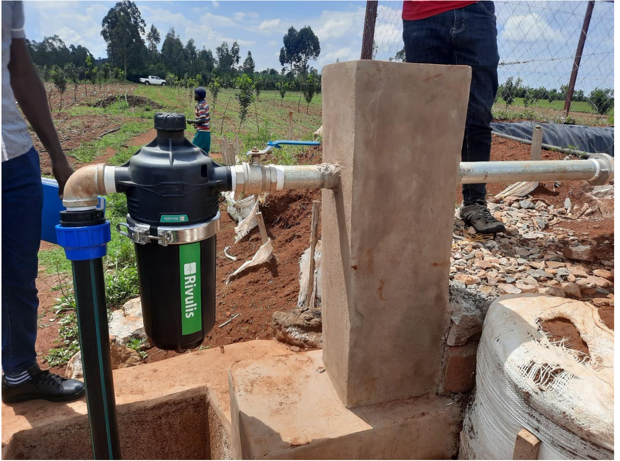
Screen filter assembly for drip irrigation system
