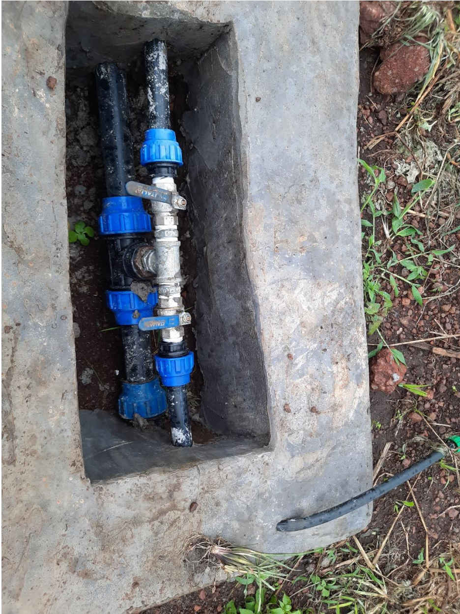
Valve assembly for 2 irrigation zones plus civil works
