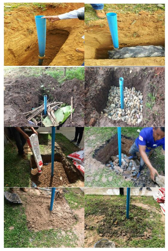
Figure 26: Closed and Recharge Wells at Surface Level Source: Netedsasanakun Water Institute
