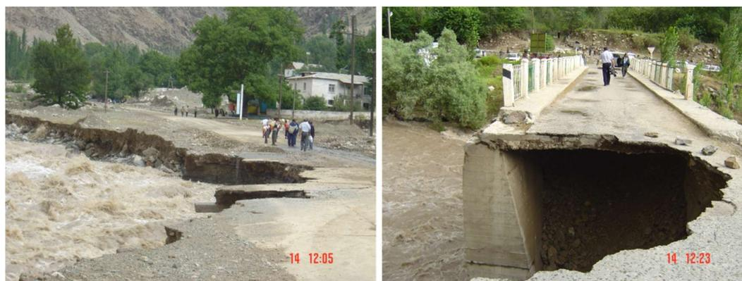
**Figure 13. Examples of damage to infrastructure in Tajikistan. Damaged road and bridge in Varzob District due to flooding and landslides after heavy rainfall. (Adapted from: ADRC country report, 2006)**
