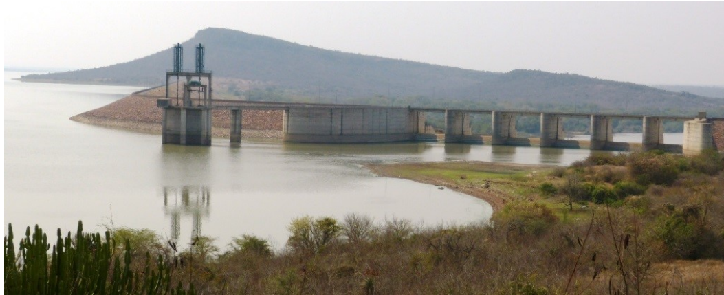
Figure 20. The sluices of Corumana reservoir ( http://www.panoramio.com/photo/96326009 )
