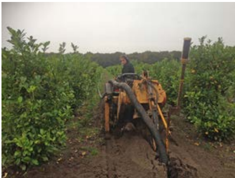
Figure 5.1 Installation of subsurface irrigation pipes
