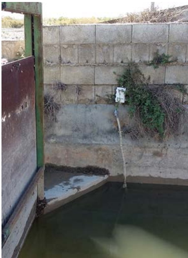
Figure 5.4 Monitoring irrigation water salinity system installed in Dalt channel
