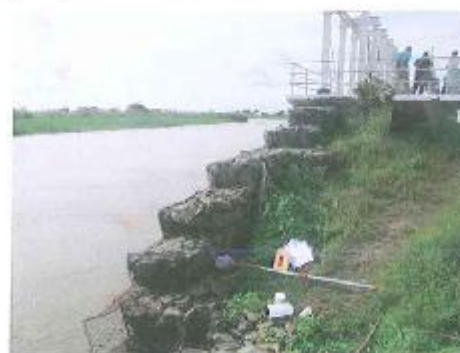
FIPAG Water Intake
